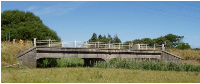
Turn of the century concrete bridge
