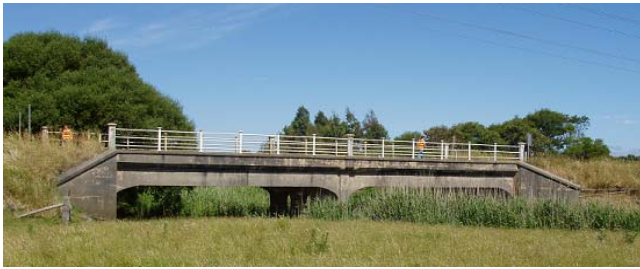
Turn of the century concrete bridge
