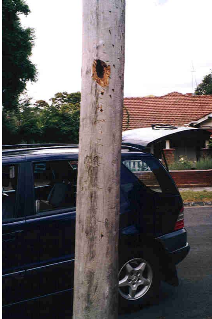
Exposed Pole from 2D result Fig:2
