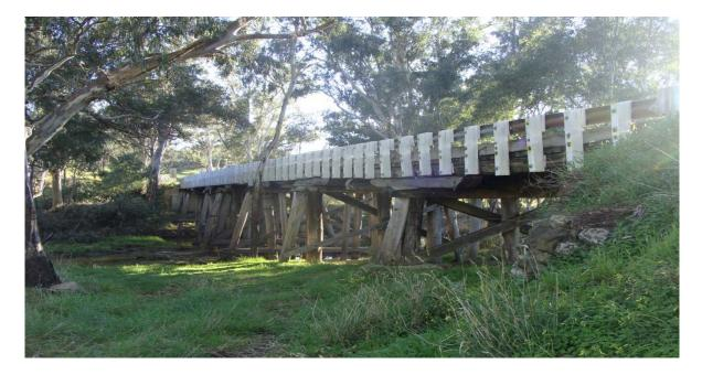
The bridge is a 50m long bridge made of rounded untreated timber subject to 100 vehicle movements per day of mixed type trucks, cars, school bus et cetera.
